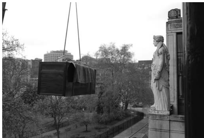
A hired crane moving furniture into its new location at No.14
